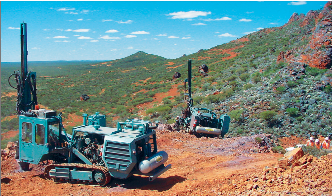
Photos front cover and above: Preparation of first bench of Talling Peak Hematite Mine, October 2003.
