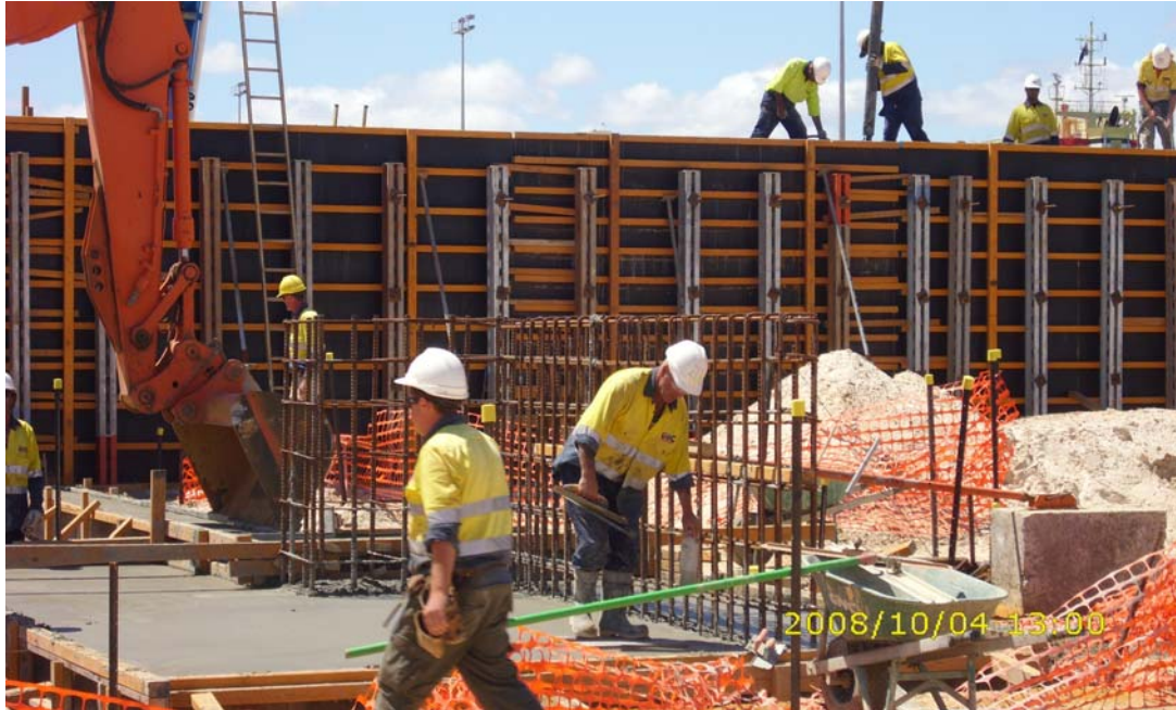
Figure 16 - Geraldton Storage Facility – Final sections of storage building walls under construction
