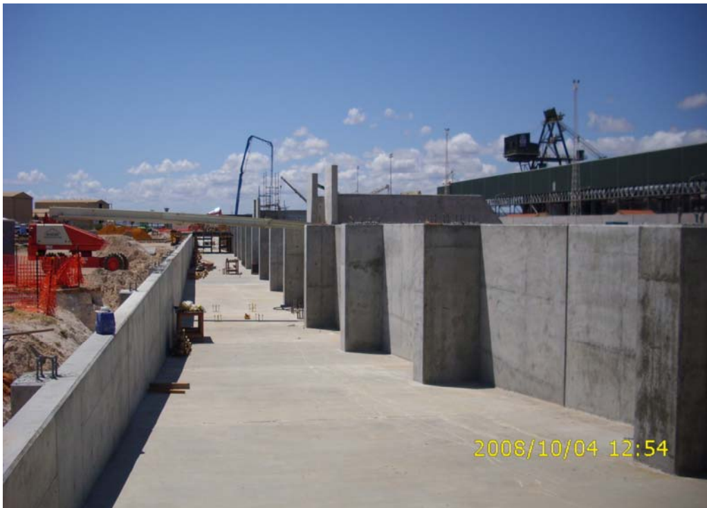
Figure 15 - Geraldton Storage Facility - Conveyor trench looking north
