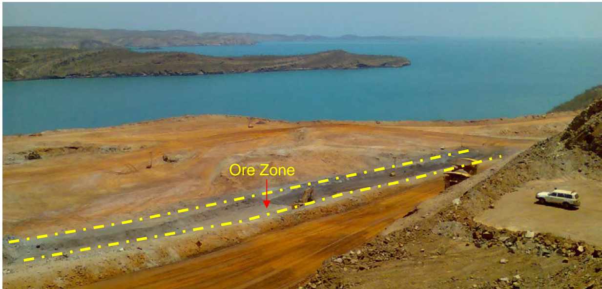
Figure 5 – Main Pit West at the end of September 2008
