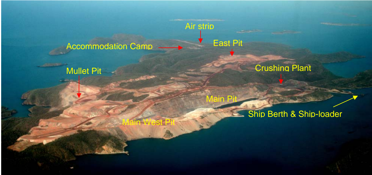
Figure 7 – Koolan Island operation at the end of September 2008
