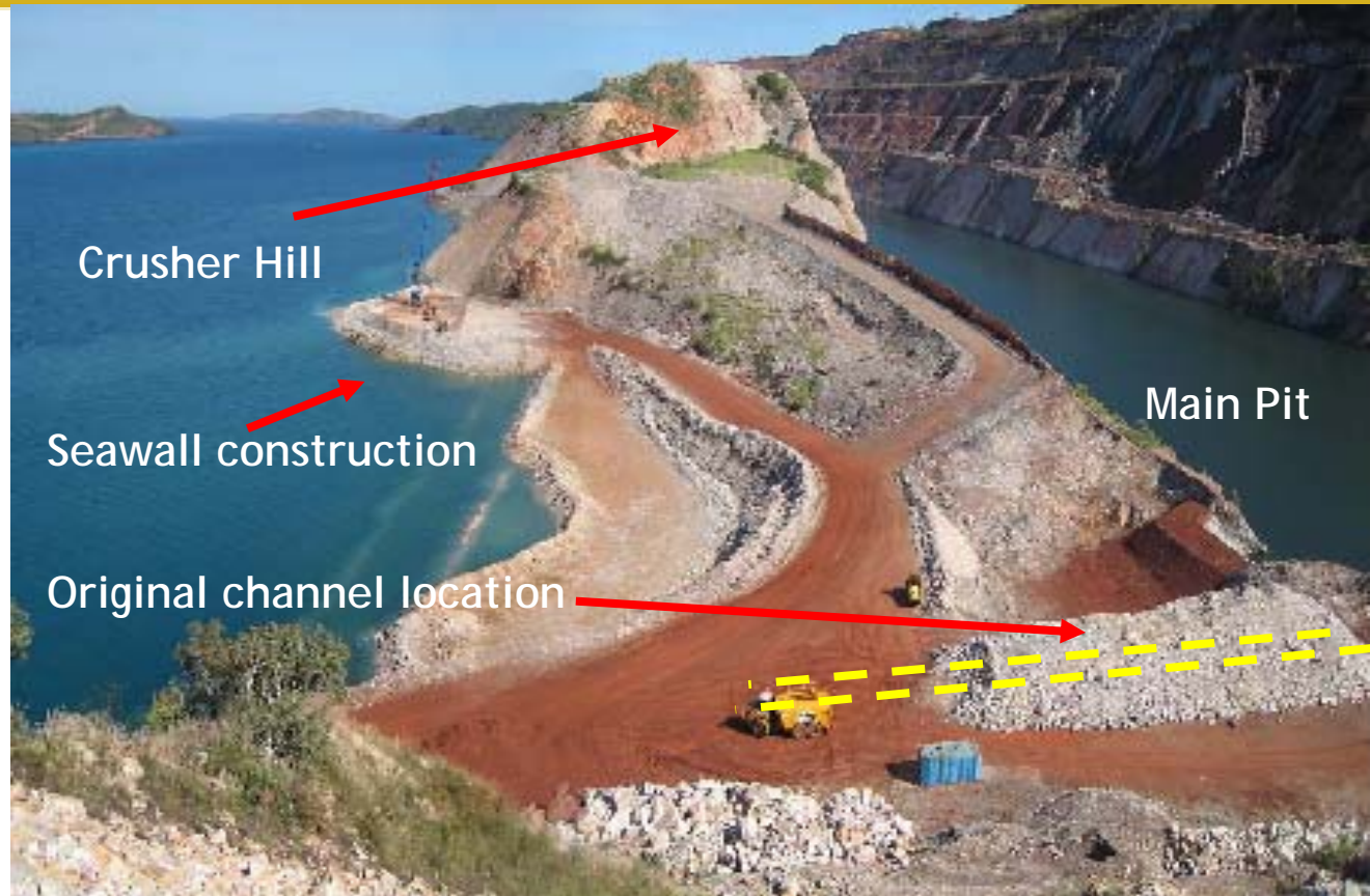
Main Pit - March 2008
