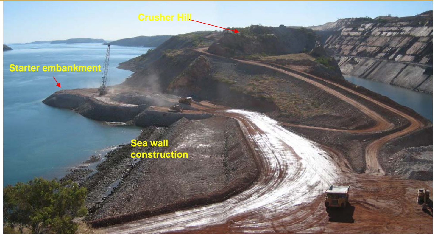
Main Pit seawall construction - June 2008
