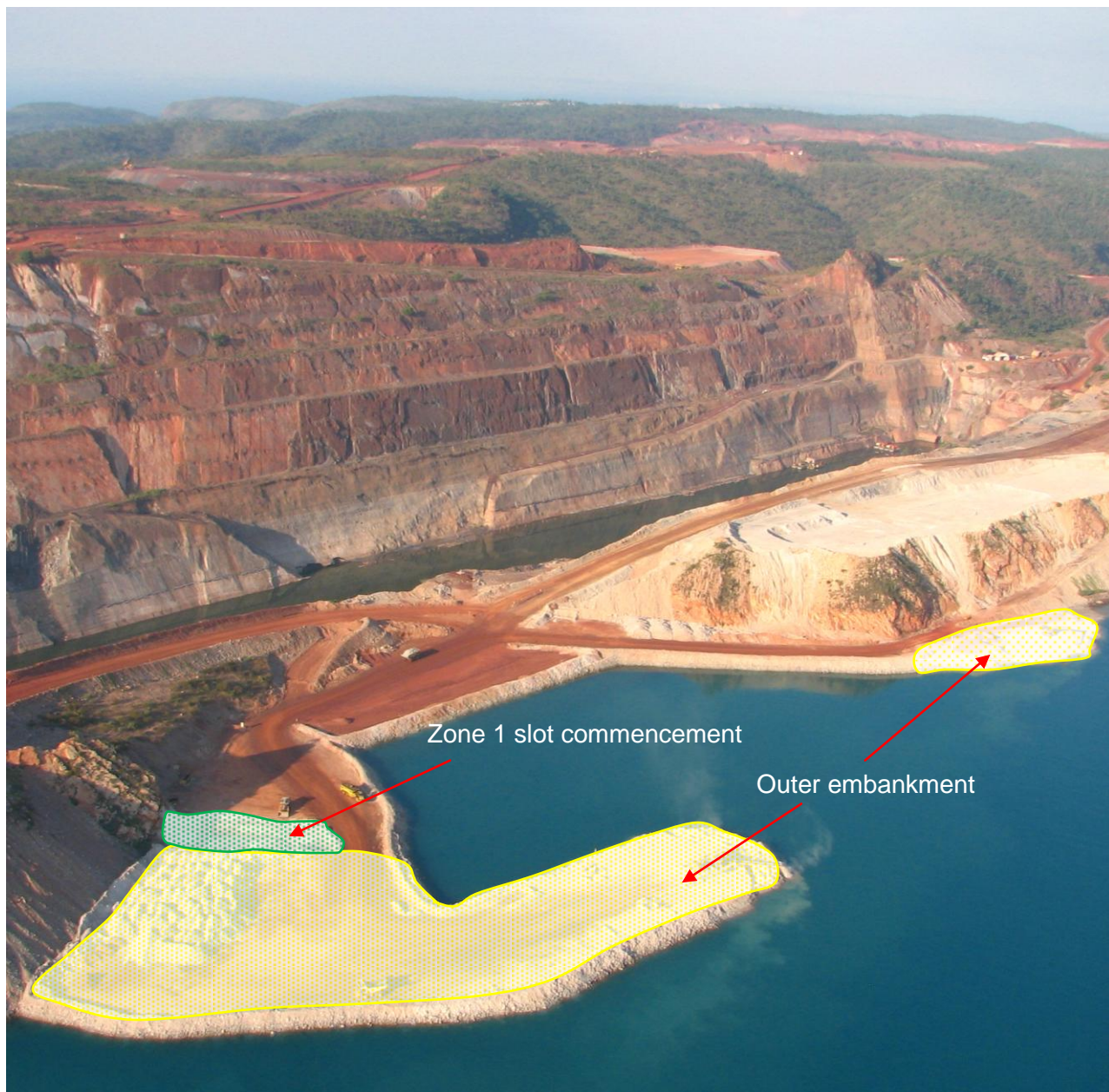
Figure 11 – Seawall outer embankment with western zone 1 slot commencing
