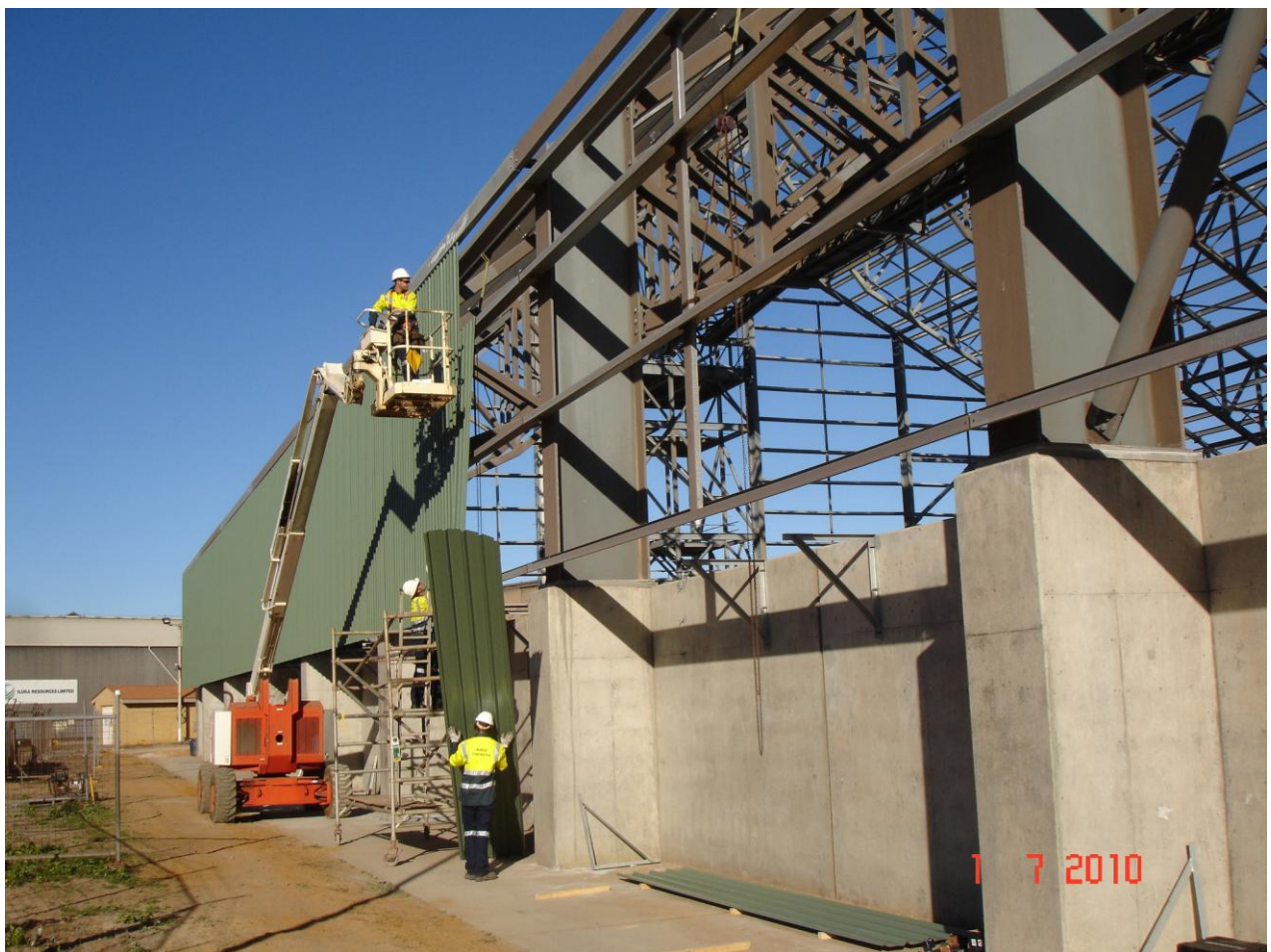
Figure 18 - Berth 5 Storage Facility cladding in progress
