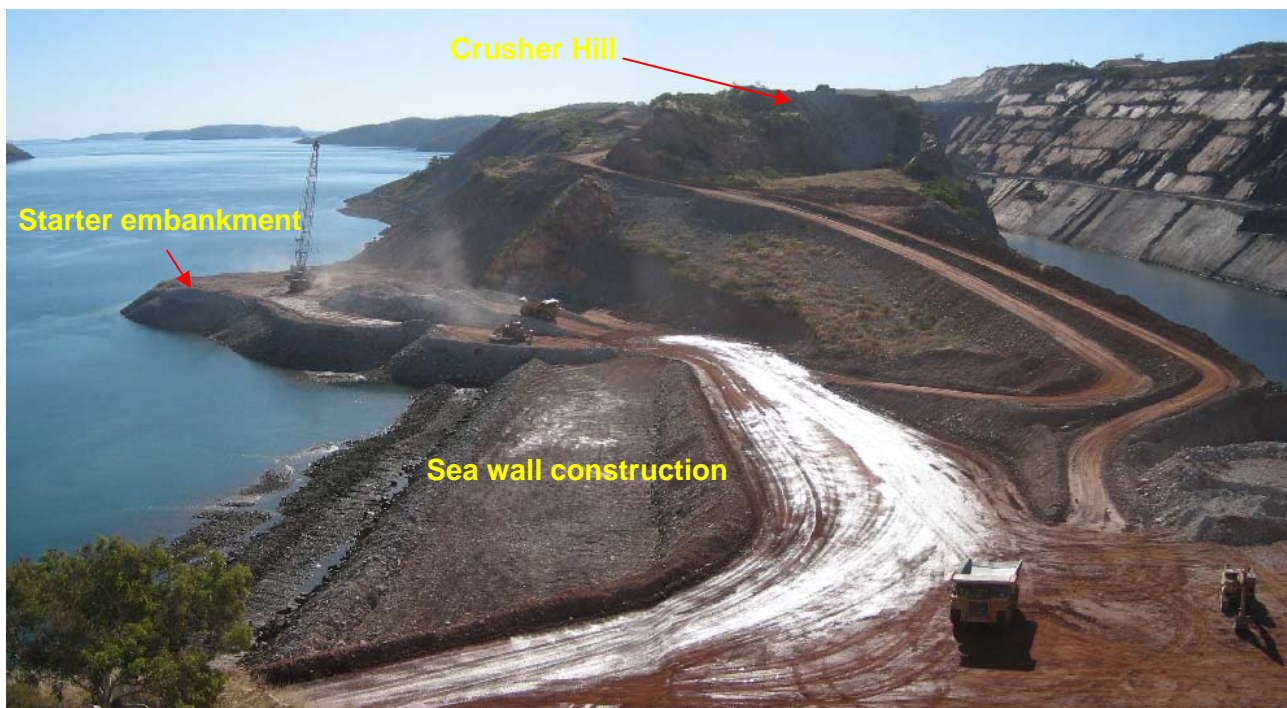
Figure 13 - Seawall & Channel plug construction looking west from Blinker Hill
