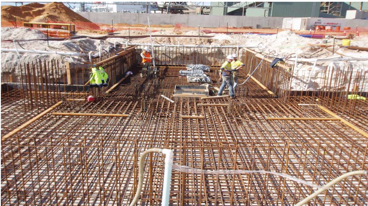
Figure 24 - Geraldton Storage Facility – Load out hopper steel fixing in progress
