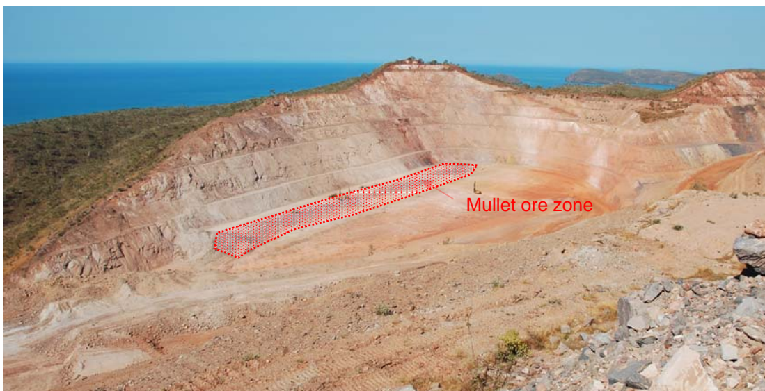
Figure 6 - Mullet Pit at the end of September 2009 showing bench development
