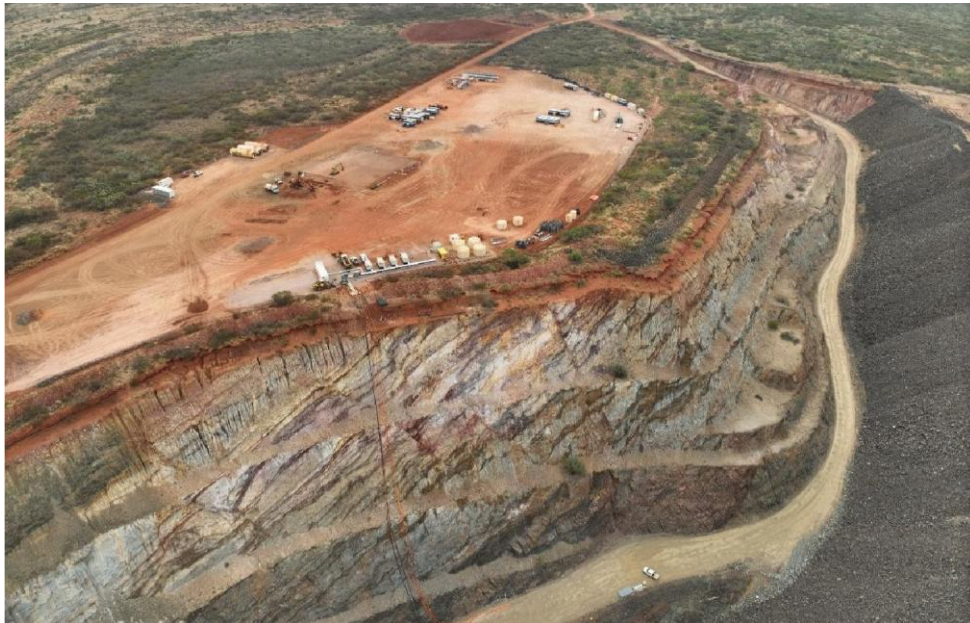
Figure 1 - Aerial view of the Groundrush open pit, looking northwest, showing the reopened pit ramp and surface infrastructure, October 2026.
