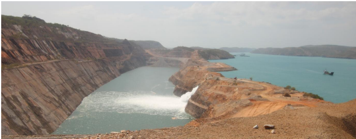
Figure 3 – Controlled flooding of the Main Pit in accordance with mine closure obligations, 27 October 2026.
