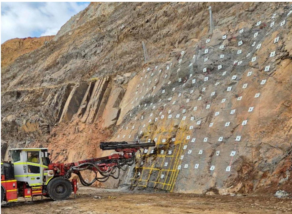
Figure 2 – Drilling for the first blast into the ventilation portal, 27 October 2026.
