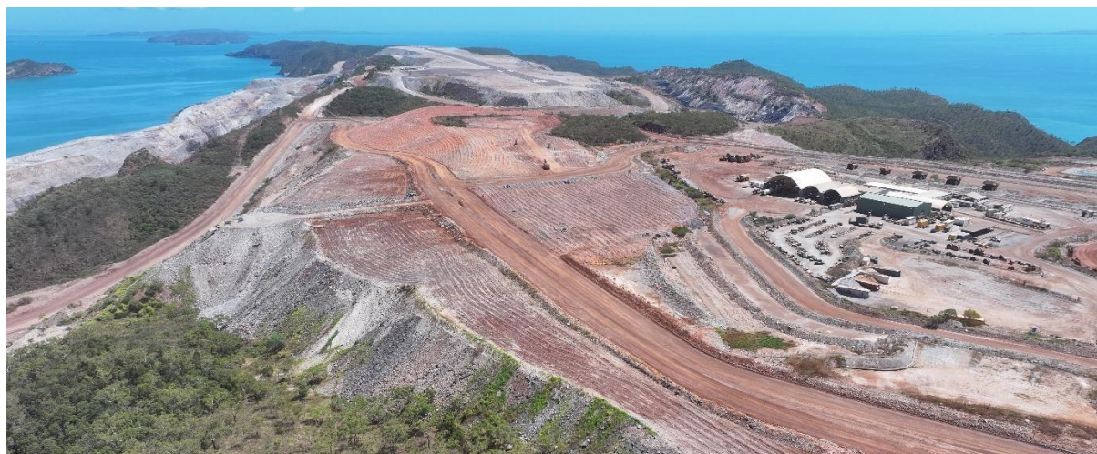
Figure 4 – Completed rehabilitation earthworks at Koolan Island, showing re-profiled, ripped and seeded areas looking west over the Mine Operations Centre and airstrip, September 2026.
