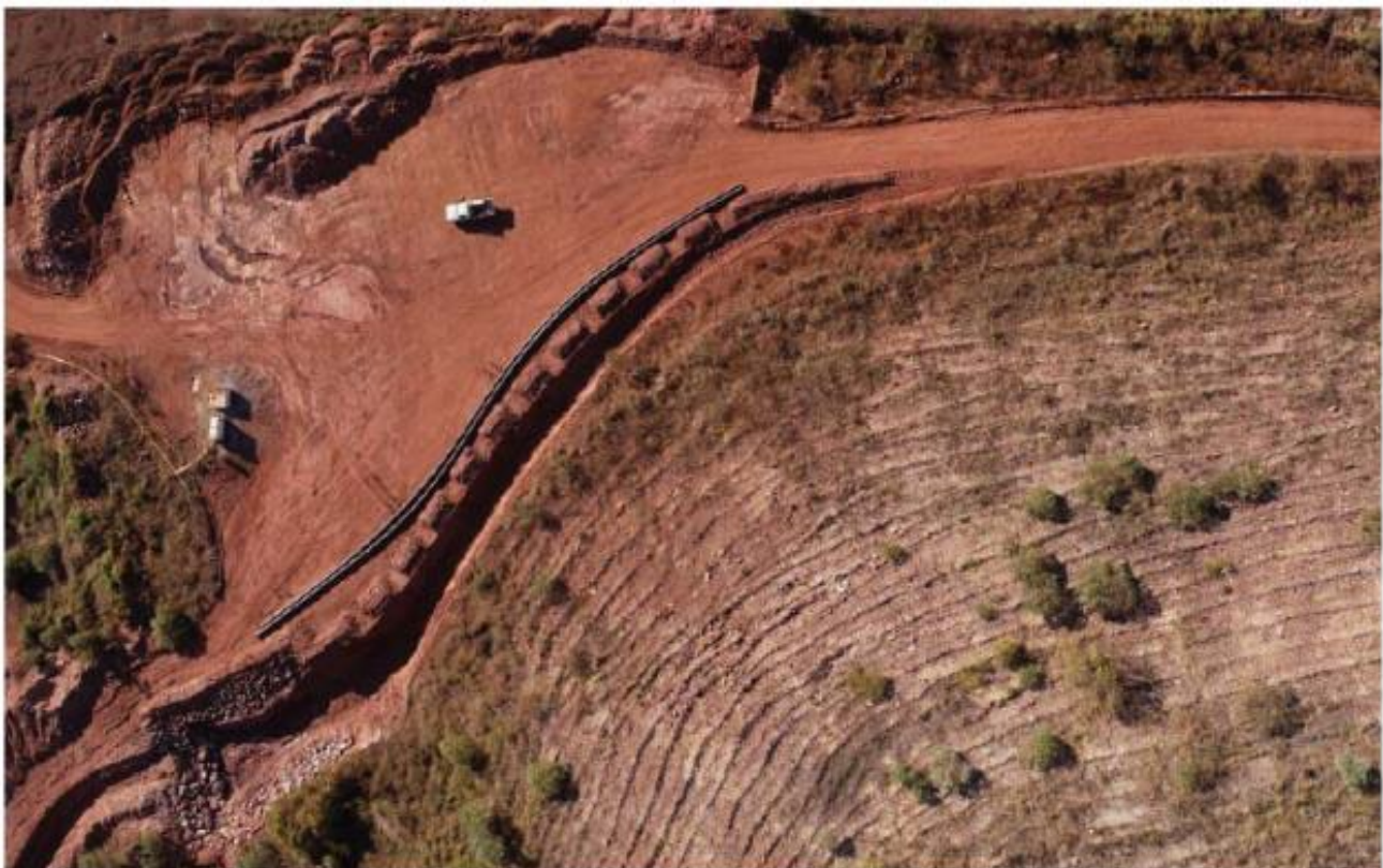
Figure 33: Drainage improvement at the crest of WD4 between waste dump lifts (July 2022). Water from runoff on upper lift is intercepted and directed away from erosive face of a lower lift.
