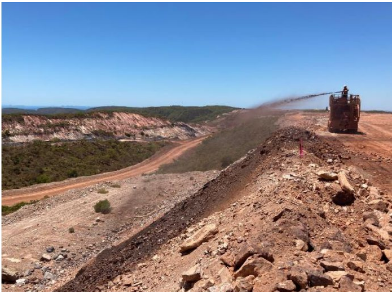
Figure 82 Hydromulch emulsion of seed in organic growth medium direct sprayed on to an angle of repose.
