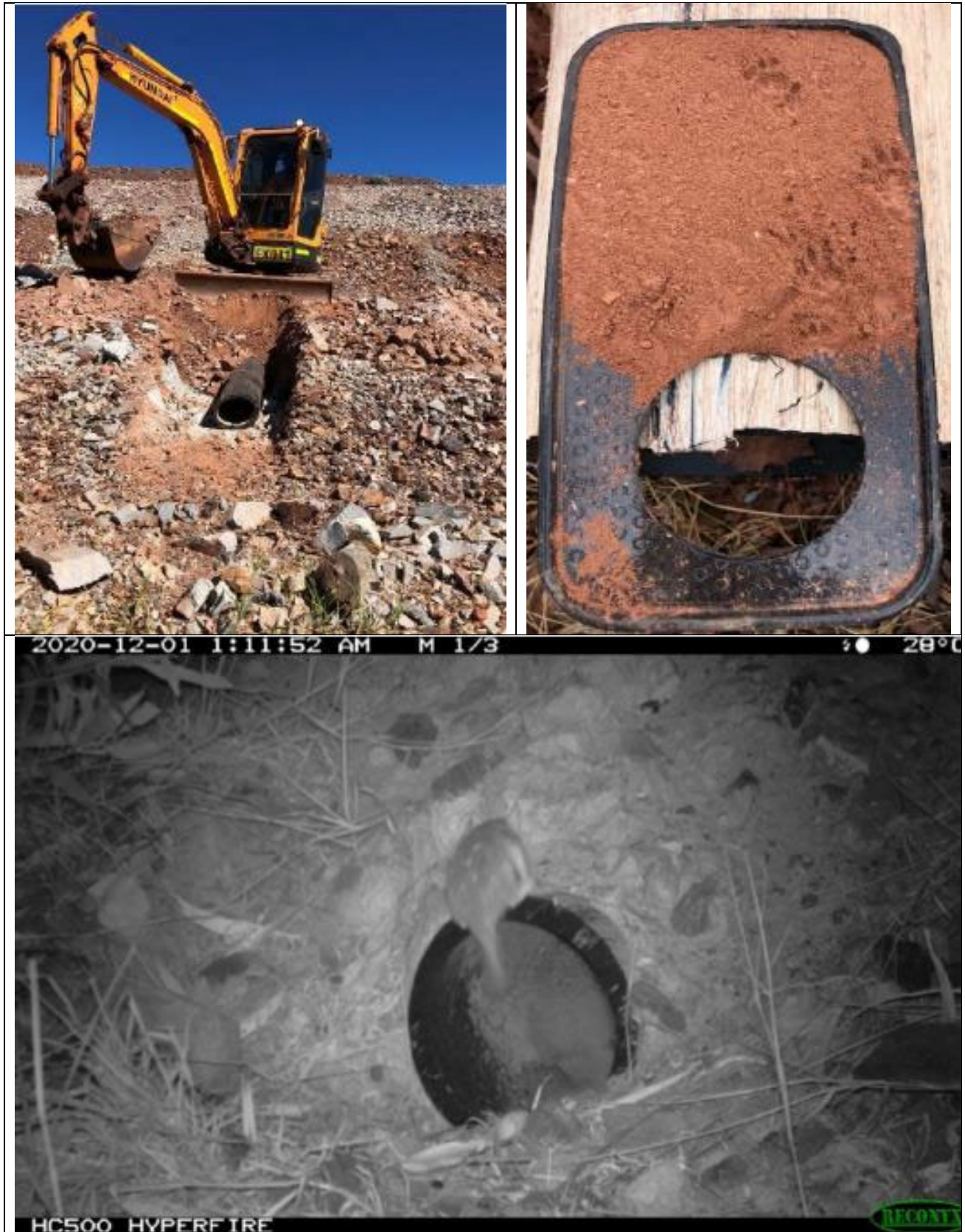
Figure 68 Installing 2m lengths of PN14 pipe (LHS); Quoll footprints at 'den' entrance (RHS). Quoll inspecting (below).
