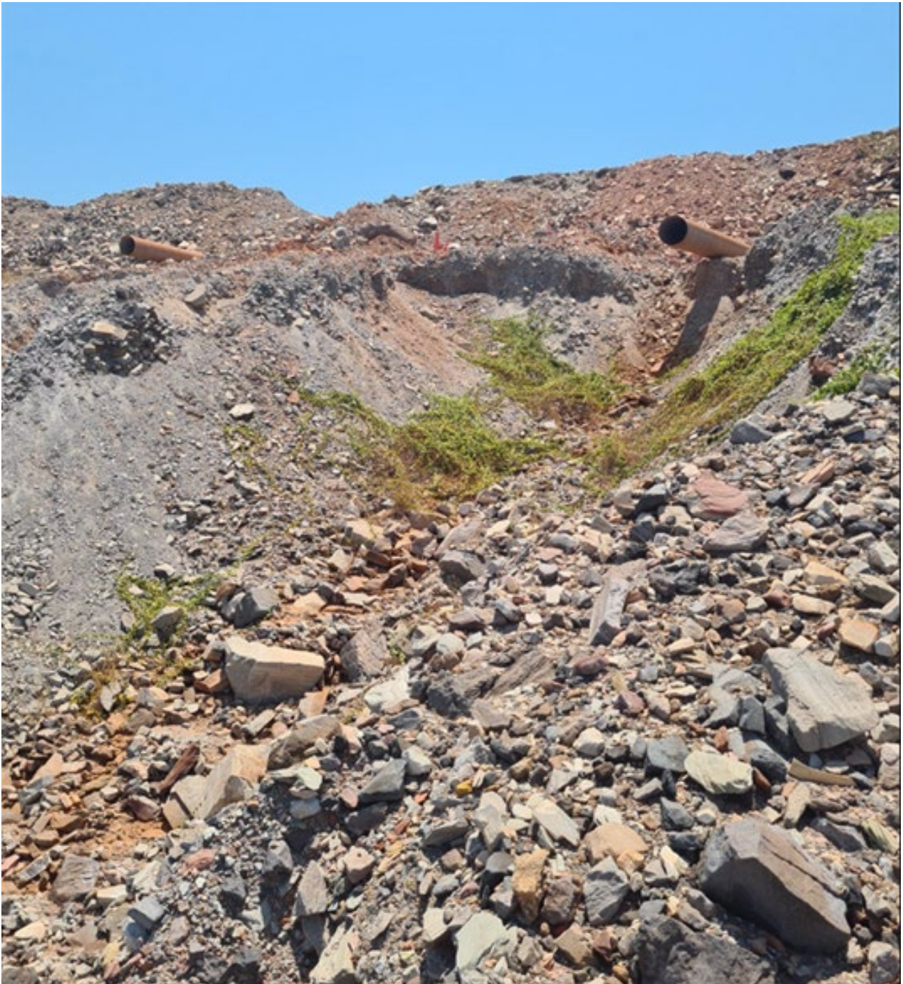
Figure 101 Erosion Feature on WD2 prior to remediation.
