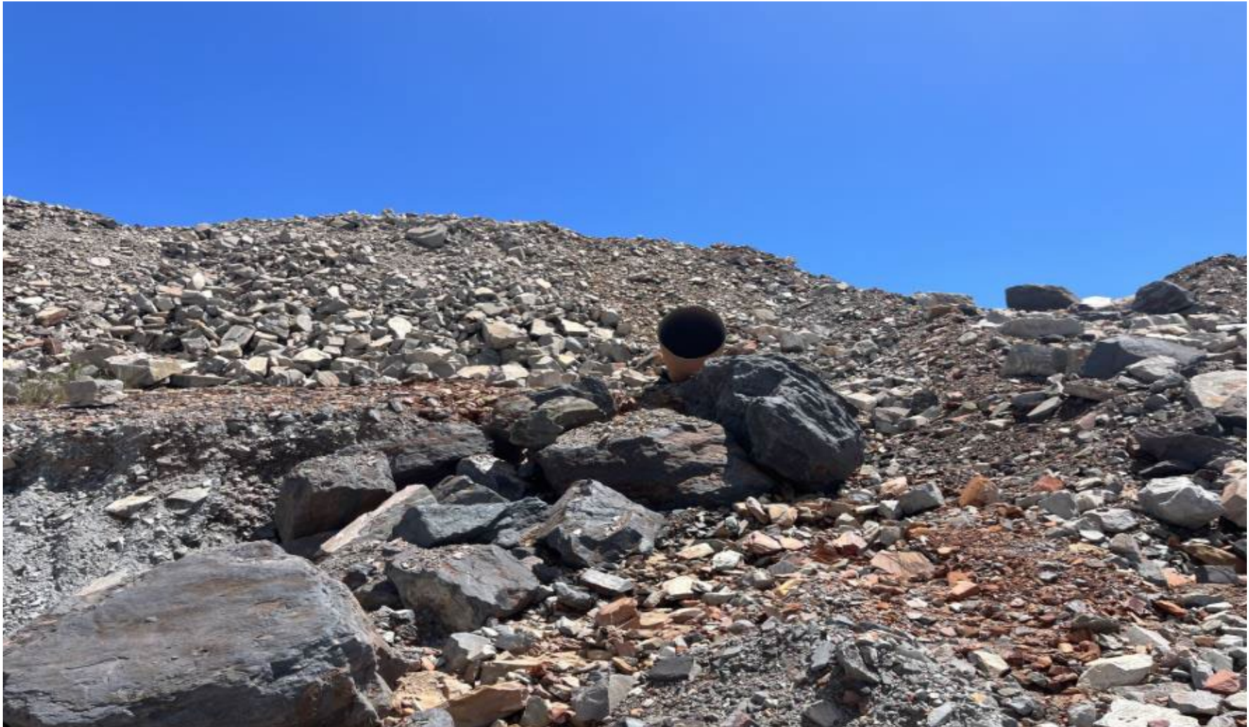
Figure 103: surface water drain after wet season (March 2024).
