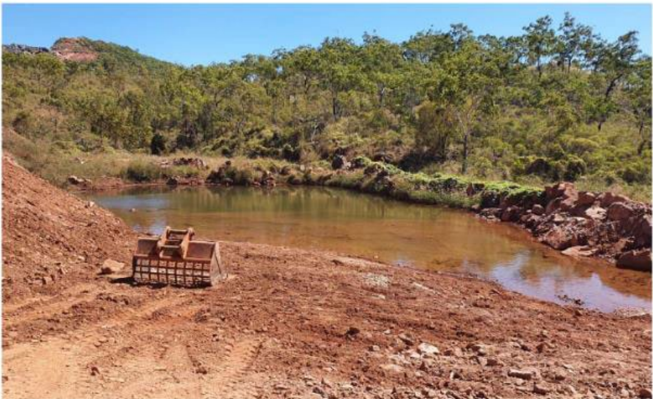
Figure 31: Drainage improvement on the bed of Pindan Creek below WD4. Earthworks to stabilise the bed and installation of rock baffles
