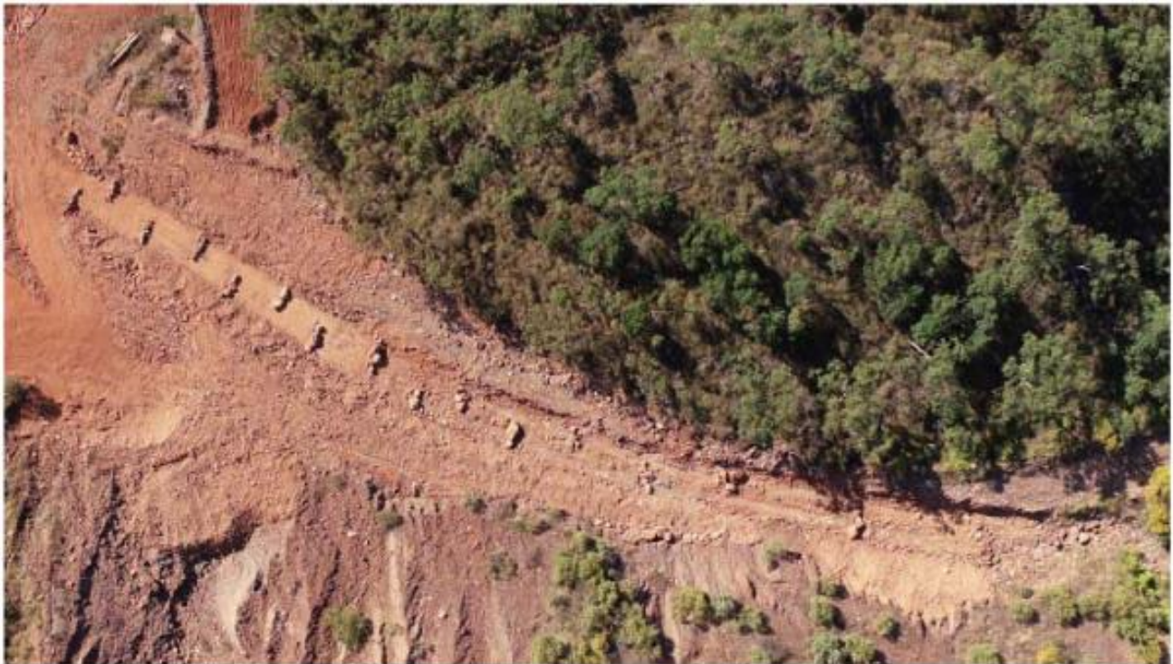
Figure 30: Sediment Trap (ST-4) after excavation of entrained sediments during 2022 dry season.
