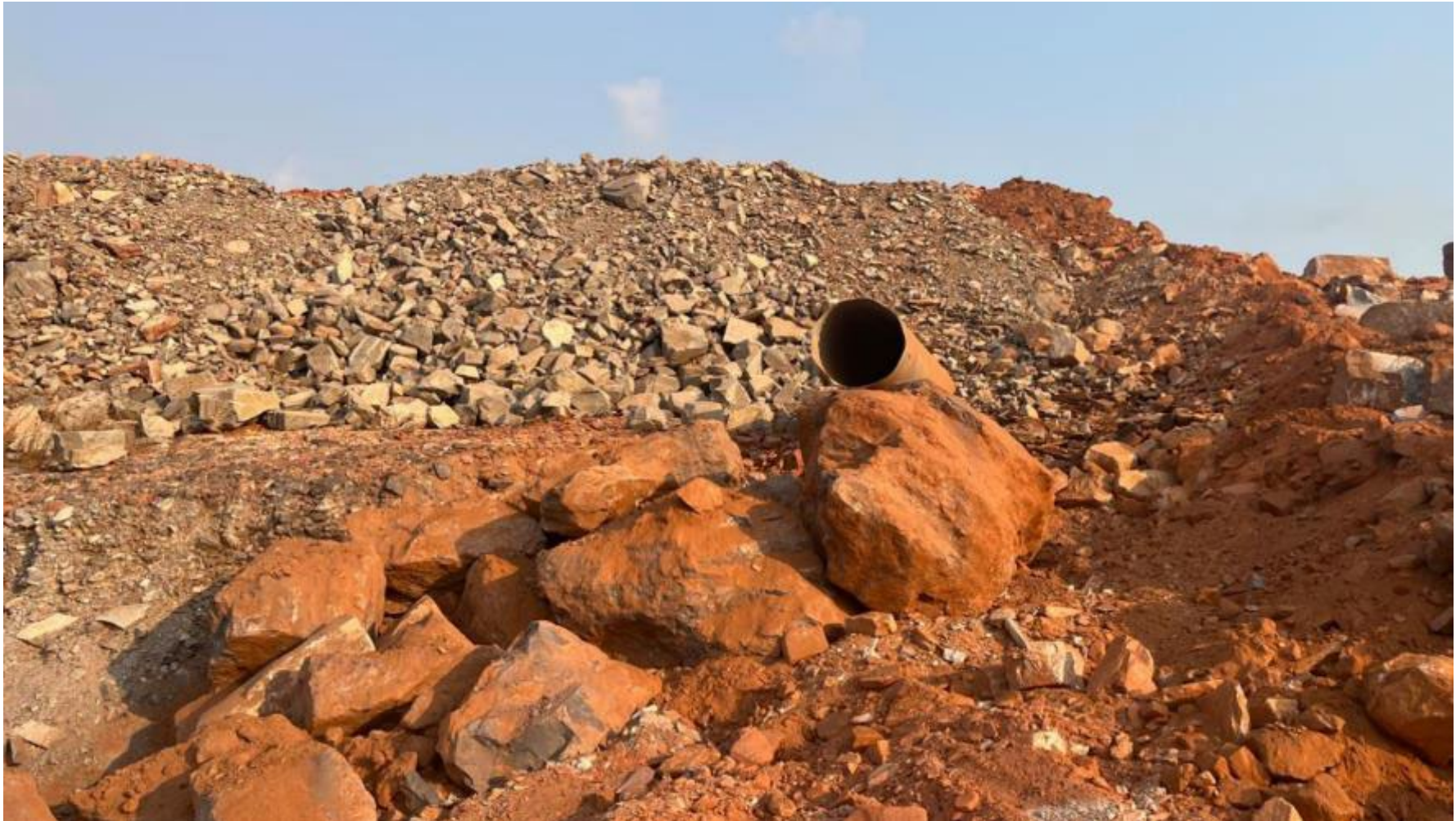
Figure 102: surface water drain after remedial works were carried out (October 2023).
