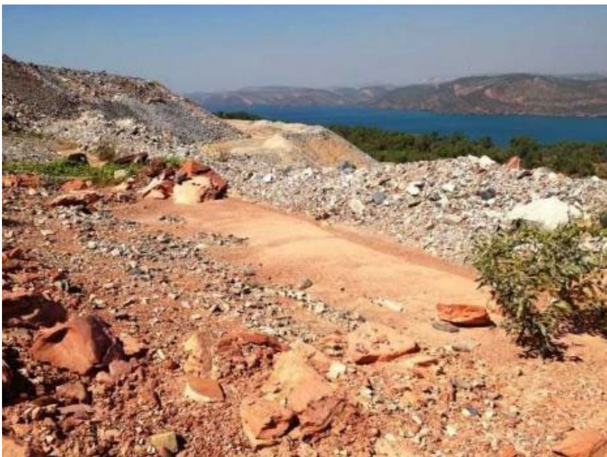
Figure 72 Accumulation of sediment on catch berm in 2015
