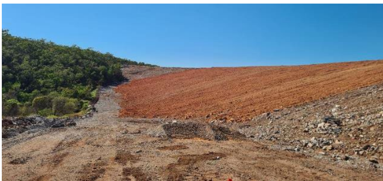
Figure 97: Final Slope Cover prior to on-contour ripping; August 2023.
