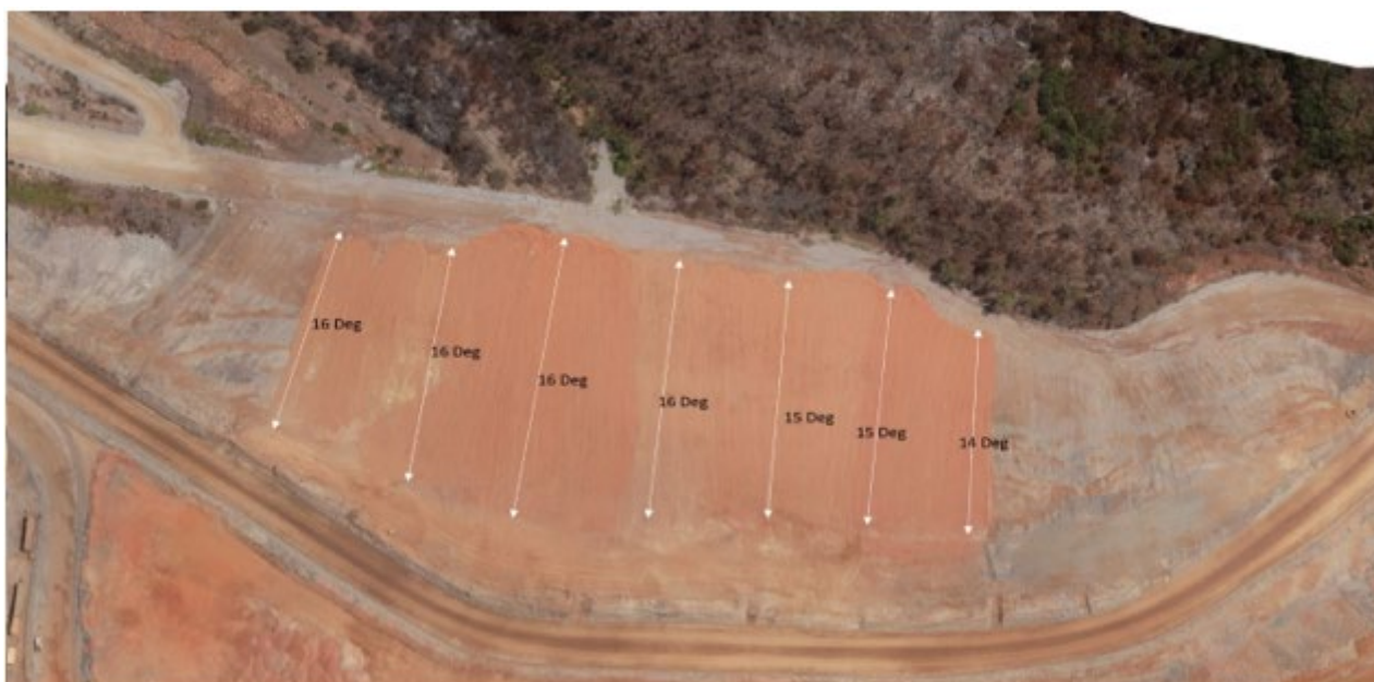
Figure 95: Capture of WRD5 showing angle of slope is <20° across the face.
