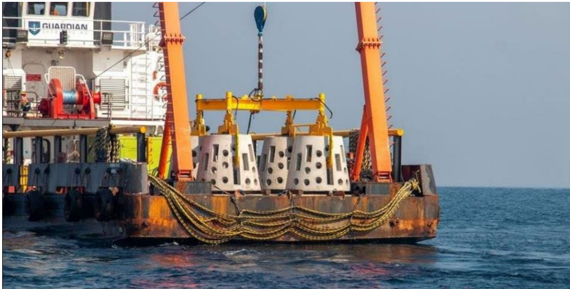
Figure 81 Example of Bombora habitat enhancement structures being installed at Ocean Reef, Perth (photo credit RecFishWest).
