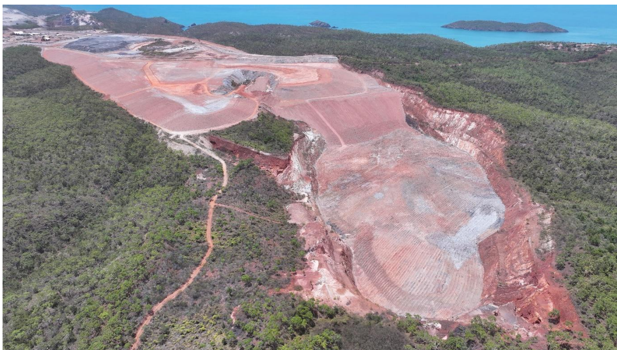
Figure 1: Rehabilitation earthworks at Koolan Island, showing final landform profiling and ripping complete ahead of seeding and the northern Australian wet season.
