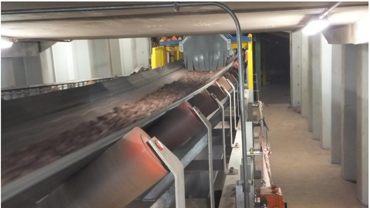
Figure 2: The new rail unloader in action.
