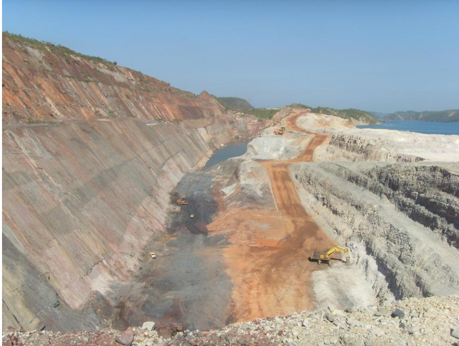
Figure 1- Pit development in Main Pit at end of March 2012, looking East.
